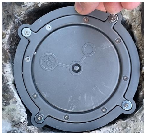
Image: Flush Mount Sensor fitting in the hole
