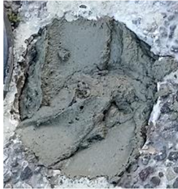
Image: Hole filled with cement
