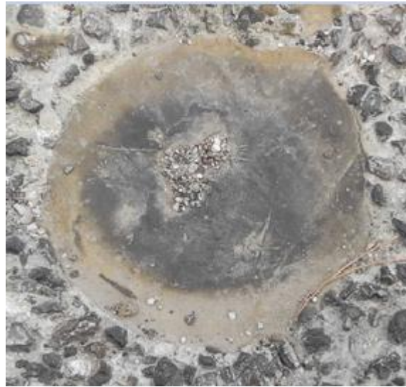
Figure-7: After the epoxy dries
