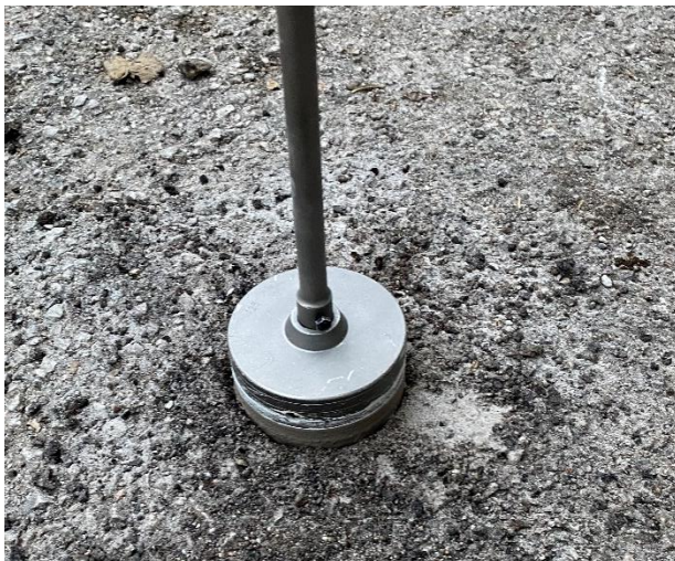
Figure-5: Drilling the hole
