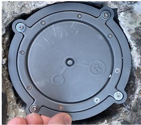
Figure-8: Flush Mount Sensor fitting in the hole
