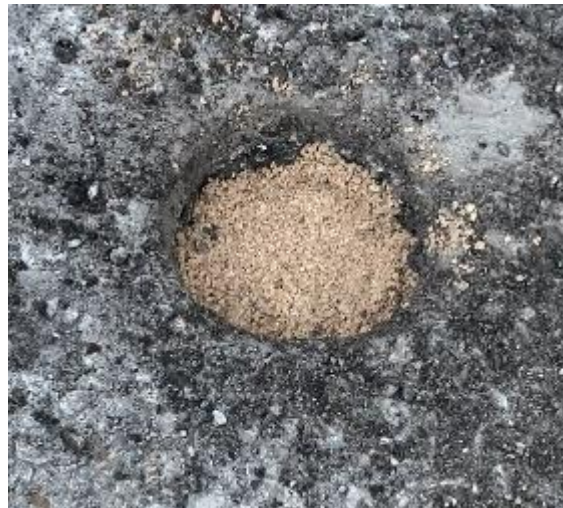
Figure-6: Placing sand in the hole
