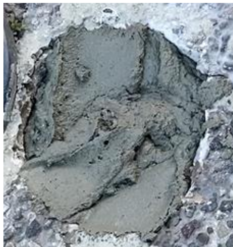
Figure-9: Hole filled with cement
